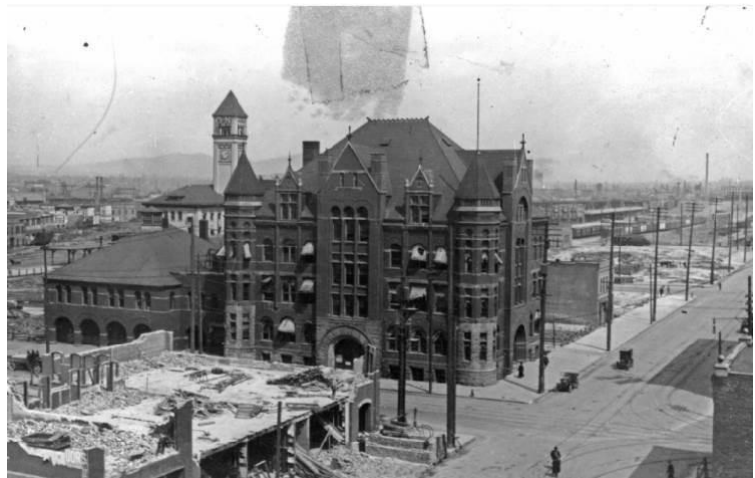
Photo of the original City Hall Building on Front (now Spokane Falls Boulevard) and Howard Street. Constructed in 1894 and demolished in 1914 for the construction of the Northern Pacific Railroad Depot (demolished for Expo '74).
